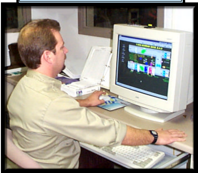
Central Alarm & Monitoring Terminal and Operator Adam
