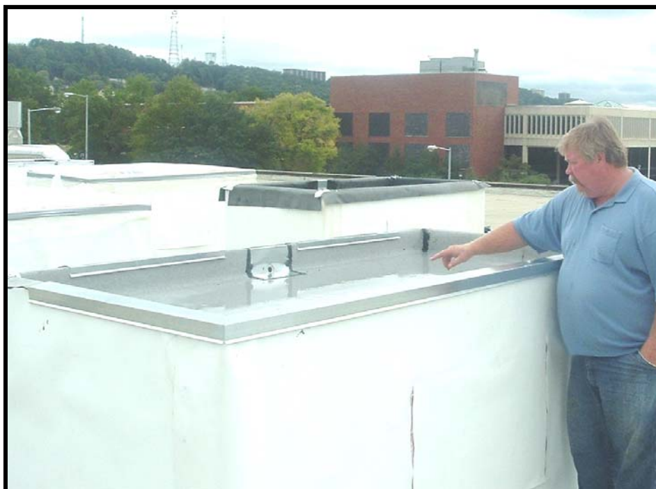
Green roof systems on the top of the Chemistry Building are currently being researched for energy conservation and sustainability.
